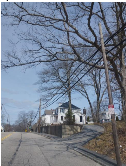
Figure 8: Tree branches intertwined with power lines, Worcester MA
