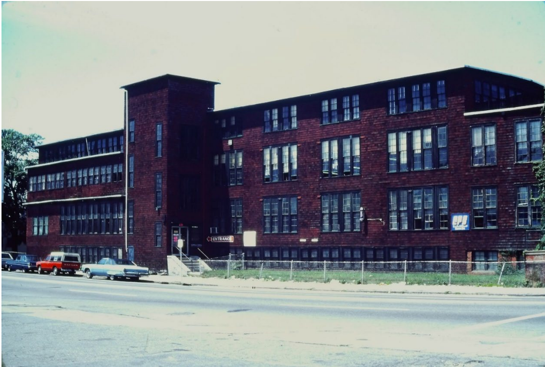
The former Worcester Slipper Company (370 Park Avenue), now the site of an Activity and Use Limitation (AUL). Source: Bmzukerman, Wikimedia.
