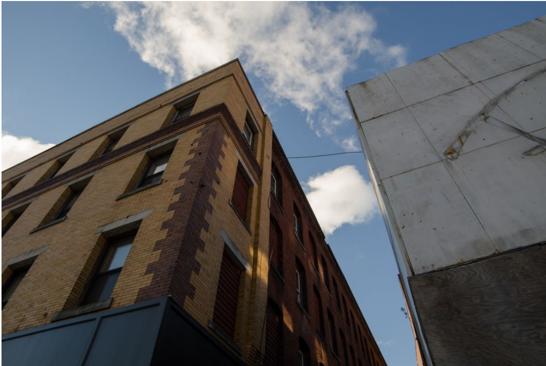
Zoning is a land use regulation that limits what can be built where. Source: Claudia Snell, Flickr.
