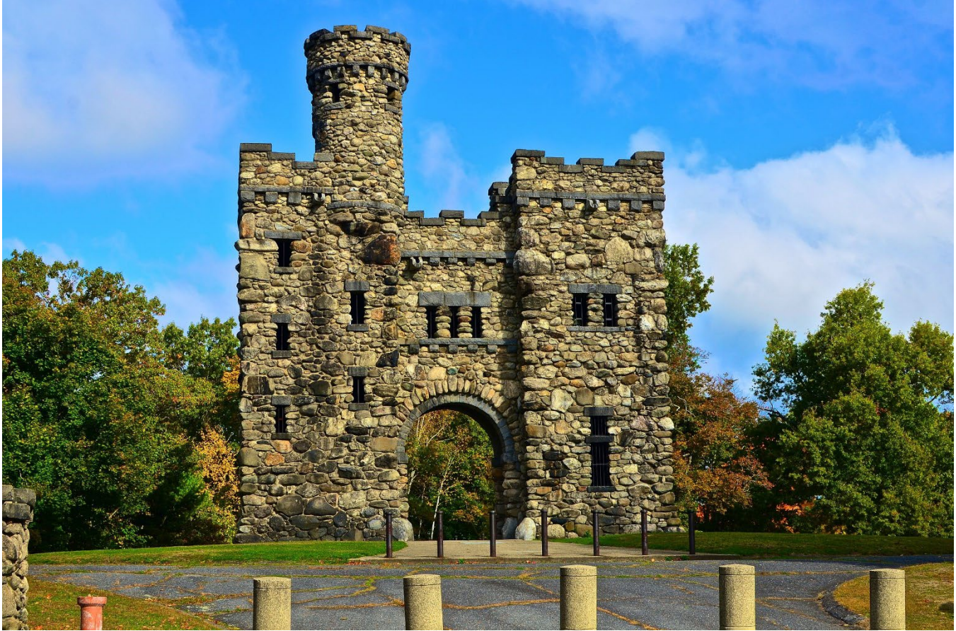
Bancroft Tower (1900), which is listed on the National Register of Historic Places. Source: Marccantlin, Wikimedia.
