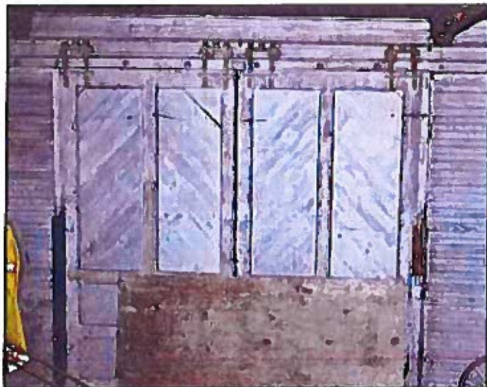
Photo 42: Original west facade main barn door with its original track and hardware remains in place behind the closed in opening. The original matched boarding that made up the panels may have been replaced with new boarding.
