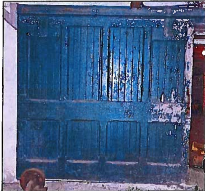
Photo 40: Door currently in the basement between the ell and the main barn is likely the original south facade main door. It has been cut down at the top to fit the basement, and may also have been reduced in width. It should be retained in its current position, but should be used as a model if a new reproduction door is made for the south facade.
