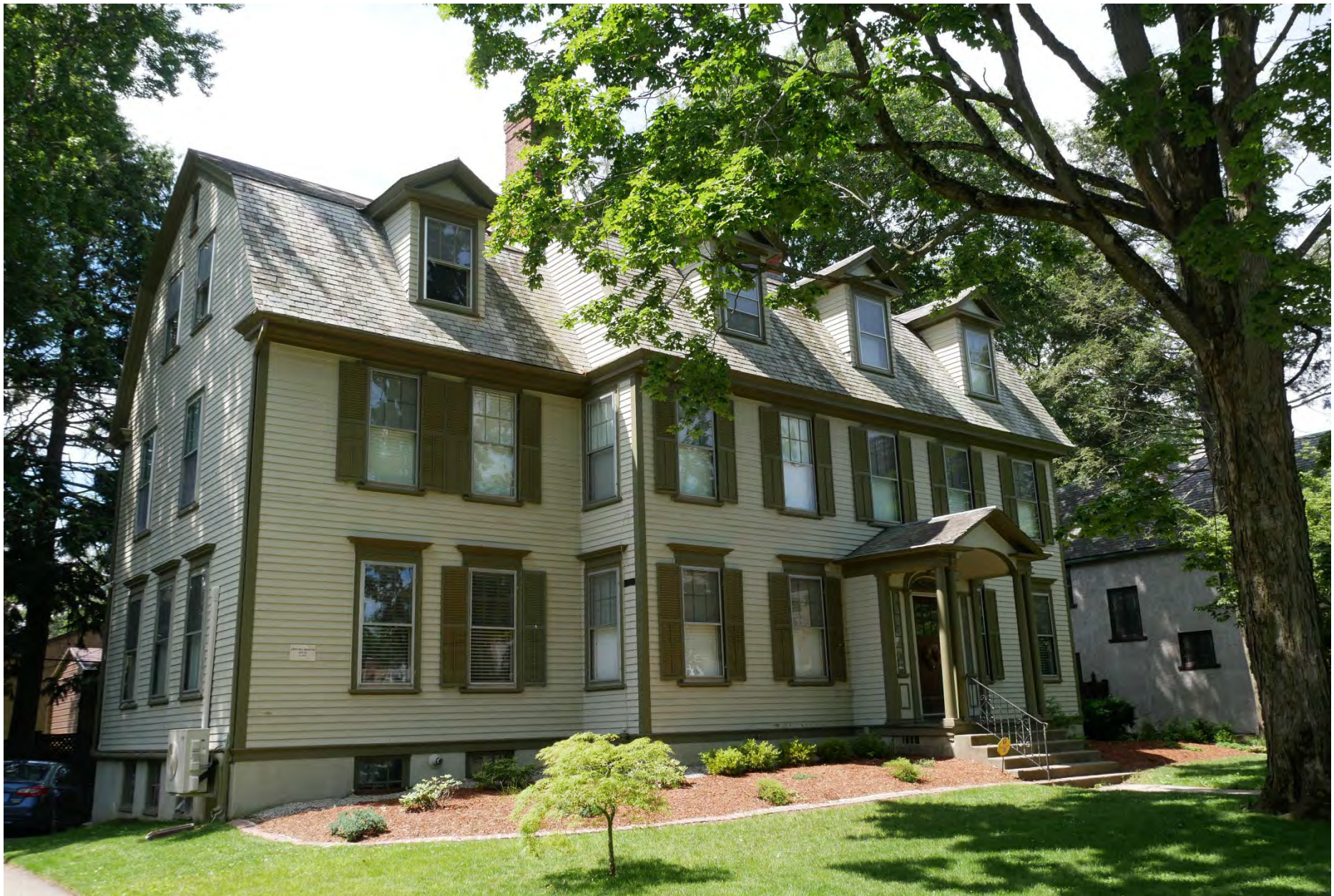
187. 85 William Street, looking southwest. Integrity rating: excellent
