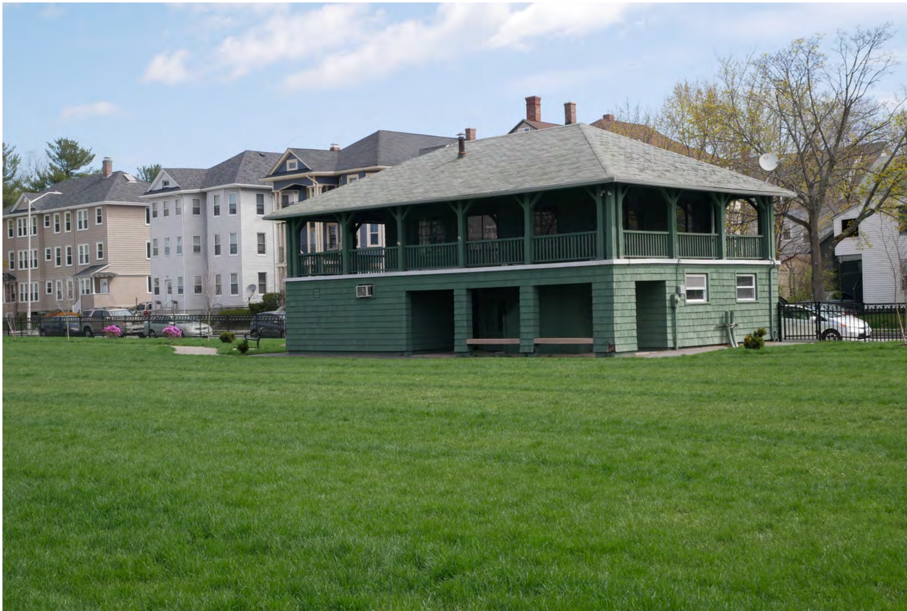
139. 69 Sever Street, looking northeast. Integrity rating: very good
