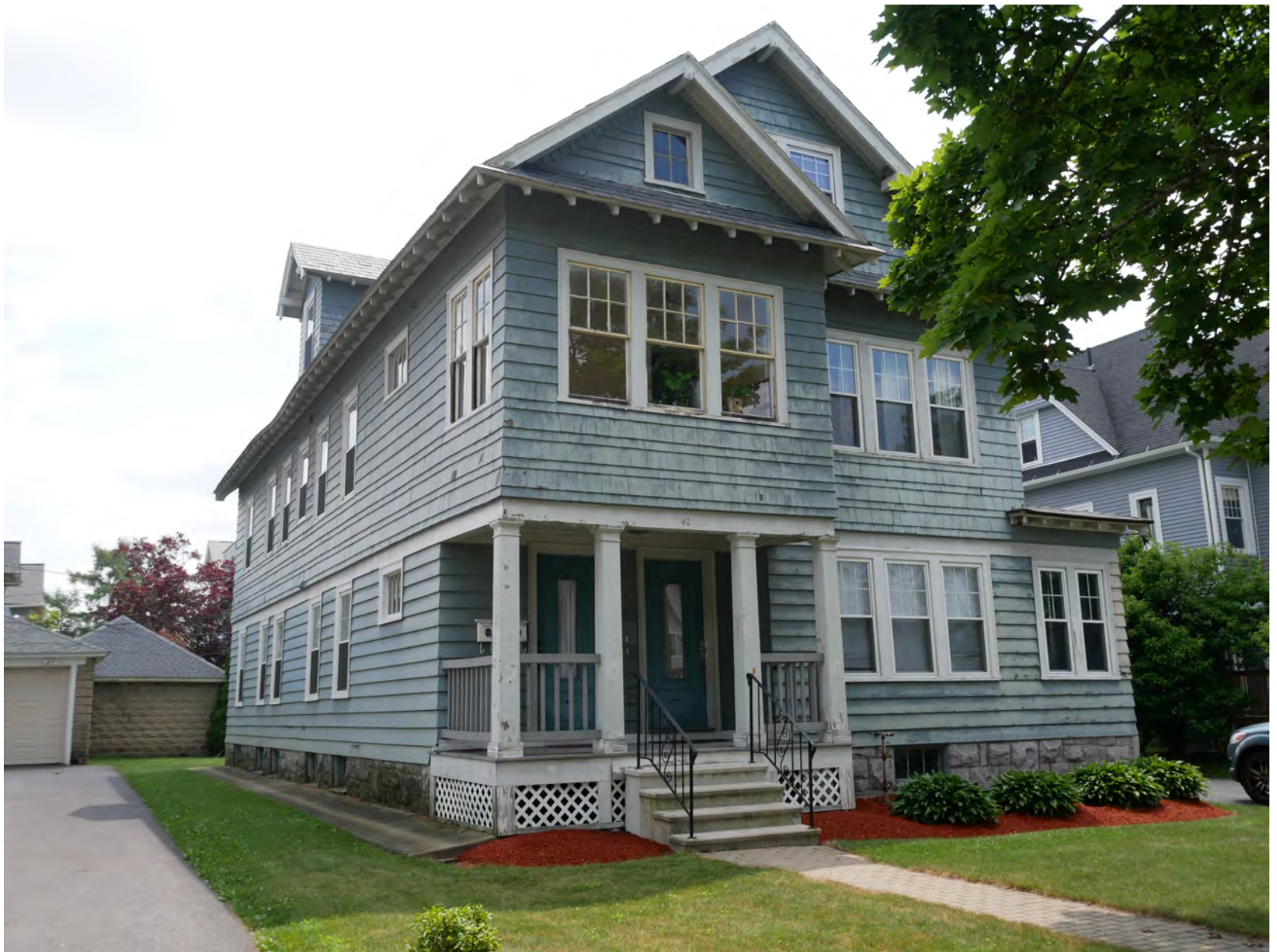
161. 42 Somerset Street, looking southeast. Integrity rating: very good
