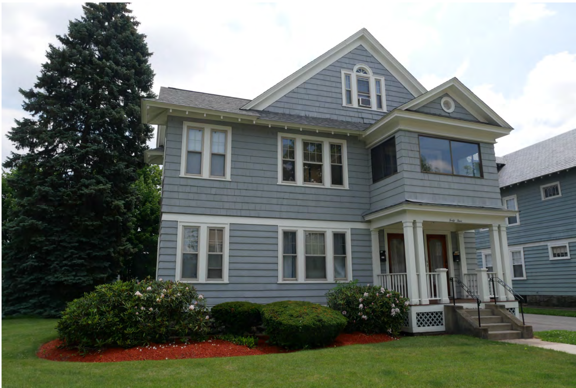
162. 44 Somerset Street, looking southeast. Integrity rating: good
