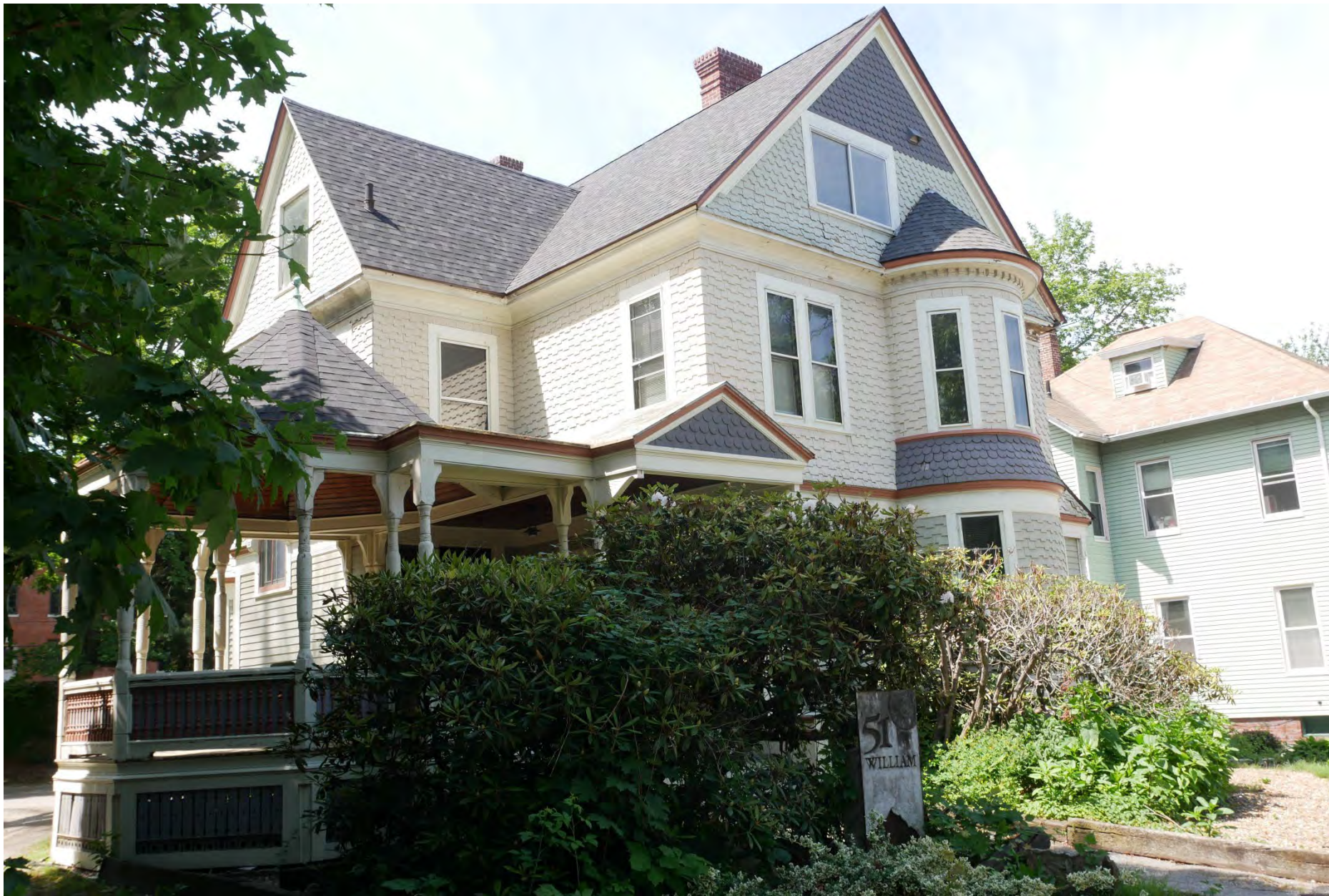
171. 51 William Street, looking southwest. Integrity rating: good
