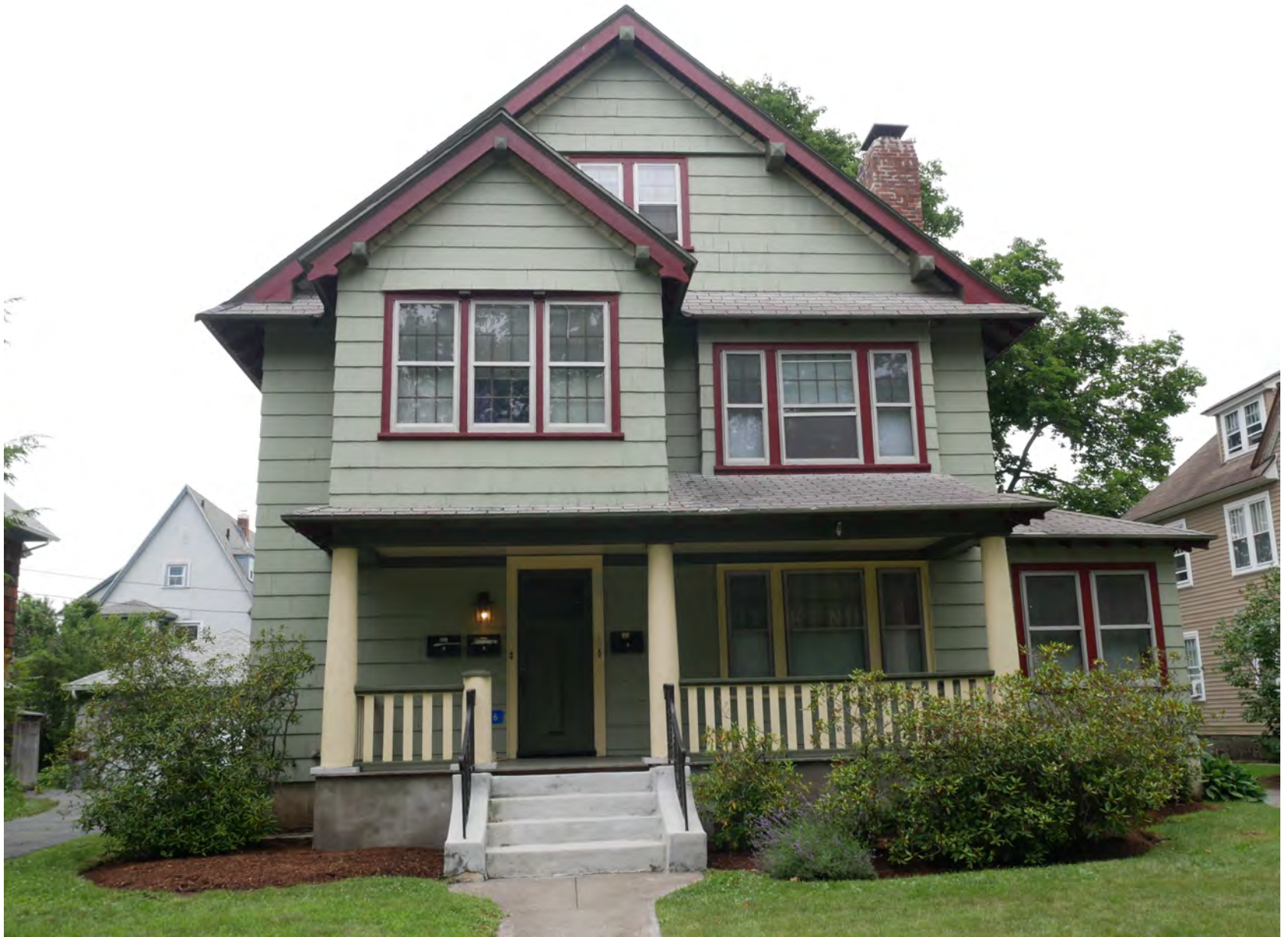
121. 156 Russell Street, looking east. Integrity rating: very good
