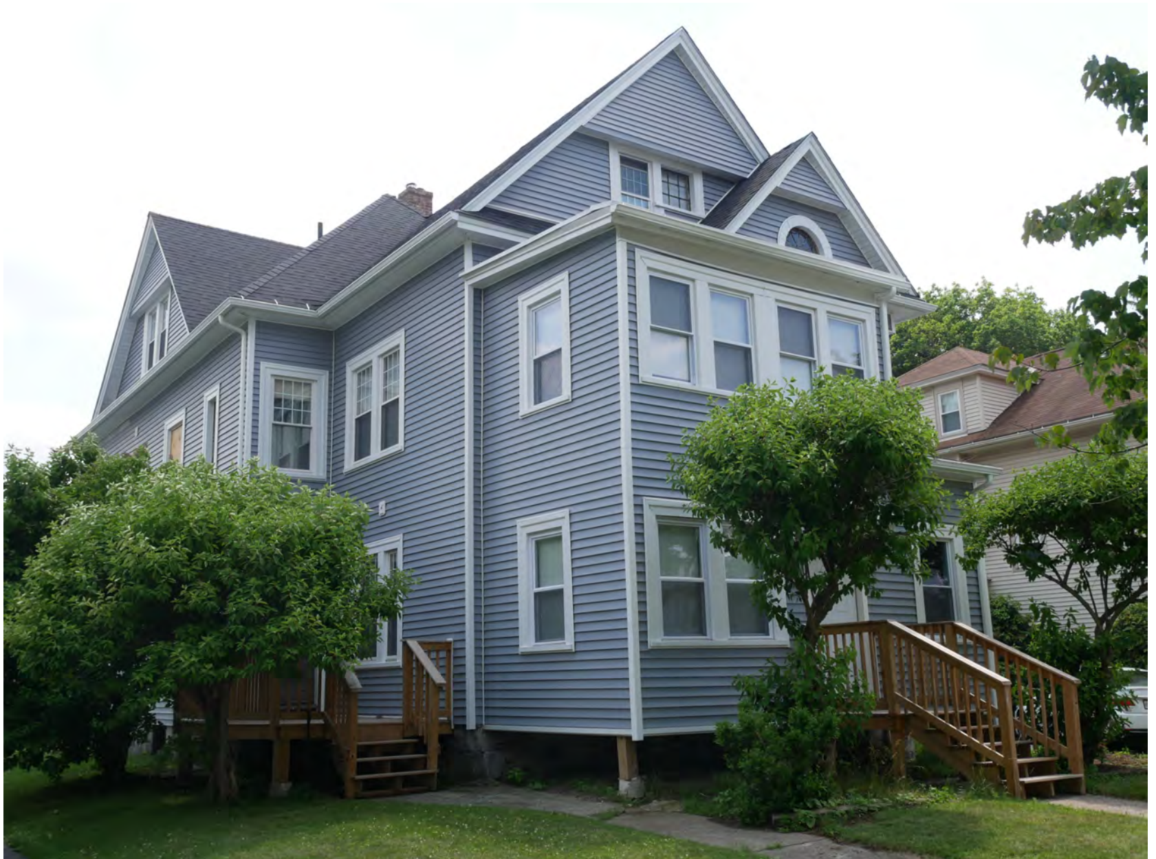
158. 36 Somerset Street, looking southeast. Integrity rating: poor
