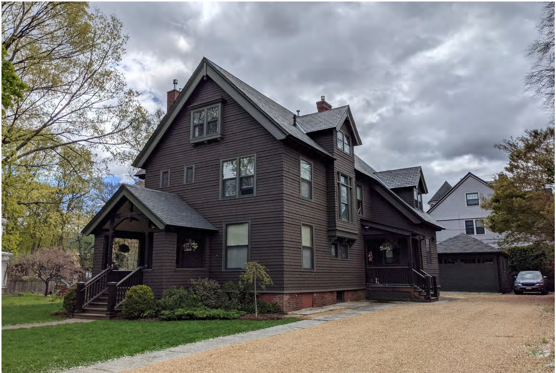
182. 79 William Street, house and garage, looking southeast. Integrity rating: very good
