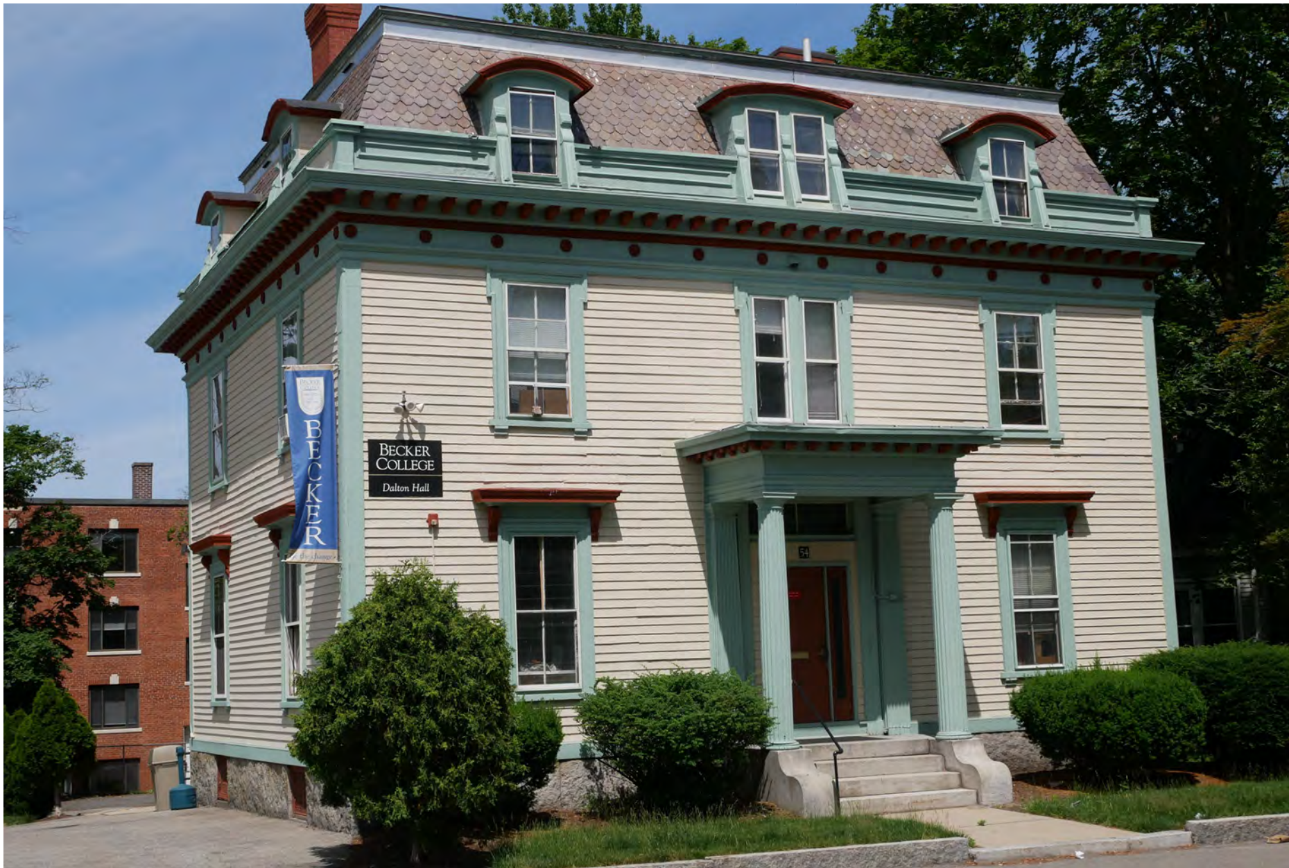
165. 54 West Street, looking northwest. Integrity rating: excellent
