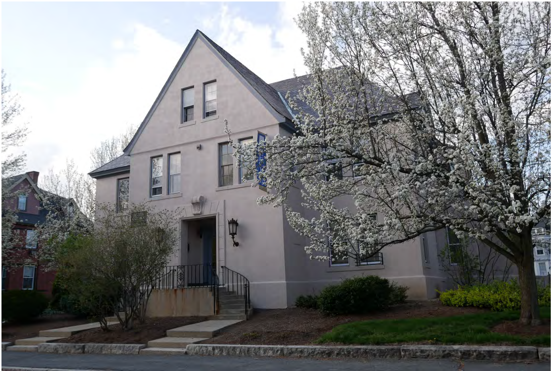
176. 60 William Street, looking northwest. Integrity rating: very good
