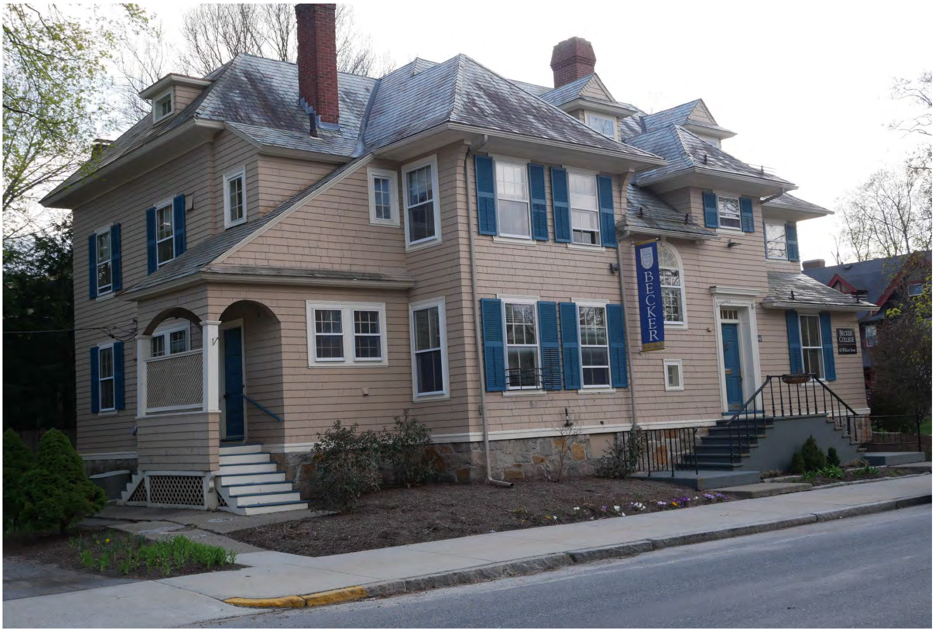
177. 61 William Street, looking southwest. Integrity rating: very good
