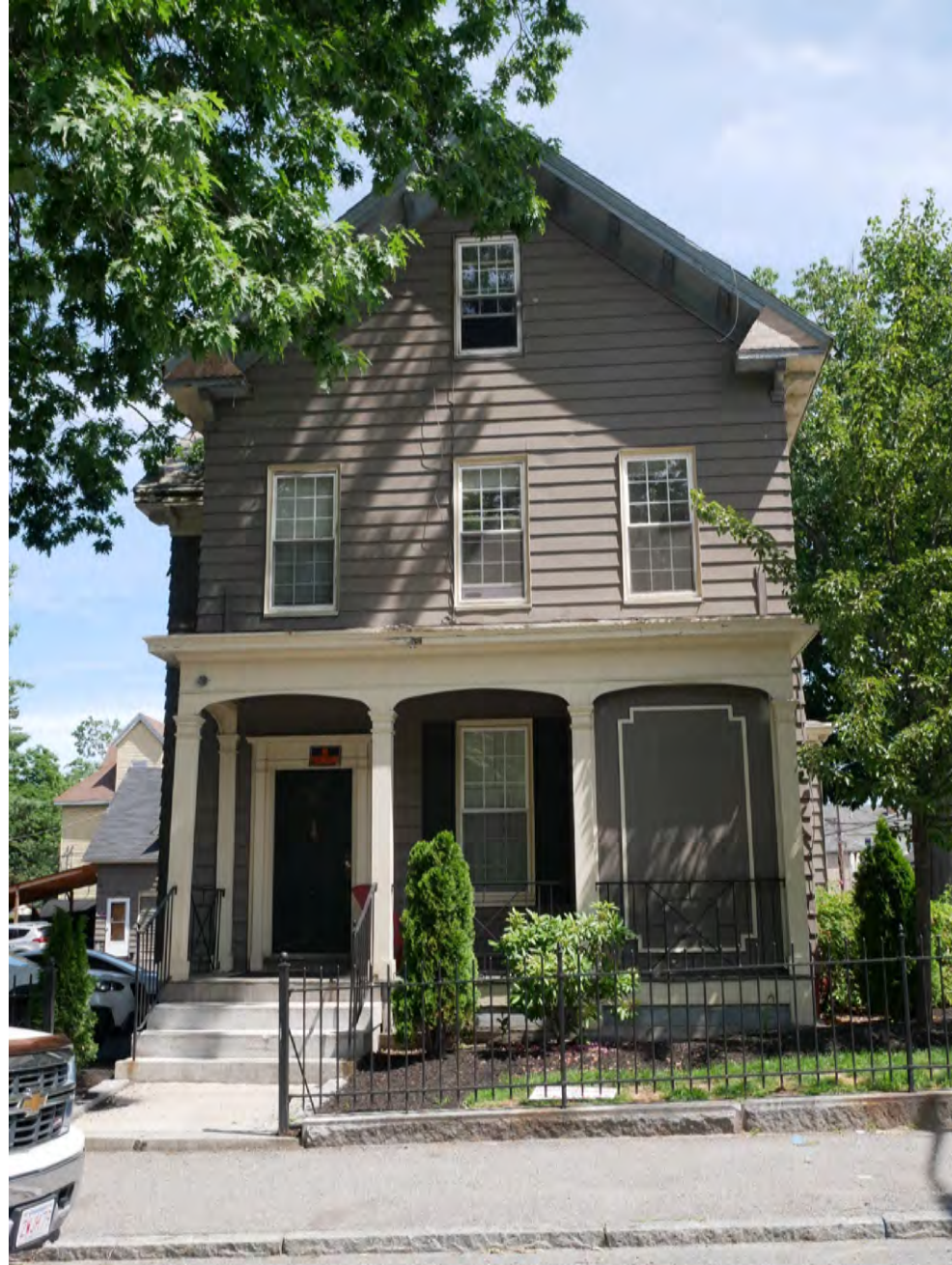
170. 50 William Street, looking north. Integrity rating: good
