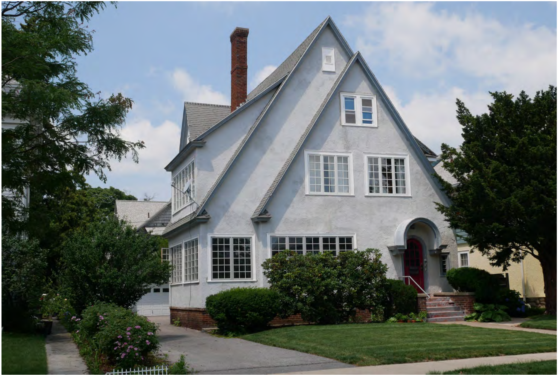
159. 37 Somerset Street, house and garage, looking northwest. Integrity rating: very good
