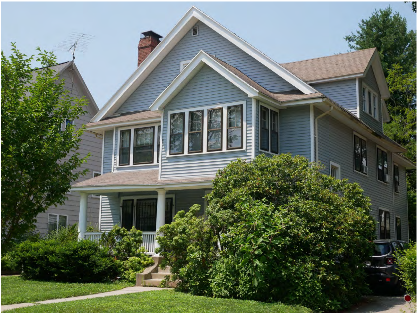
141. 9 Somerset Street, looking southwest. Integrity rating: fair to good
