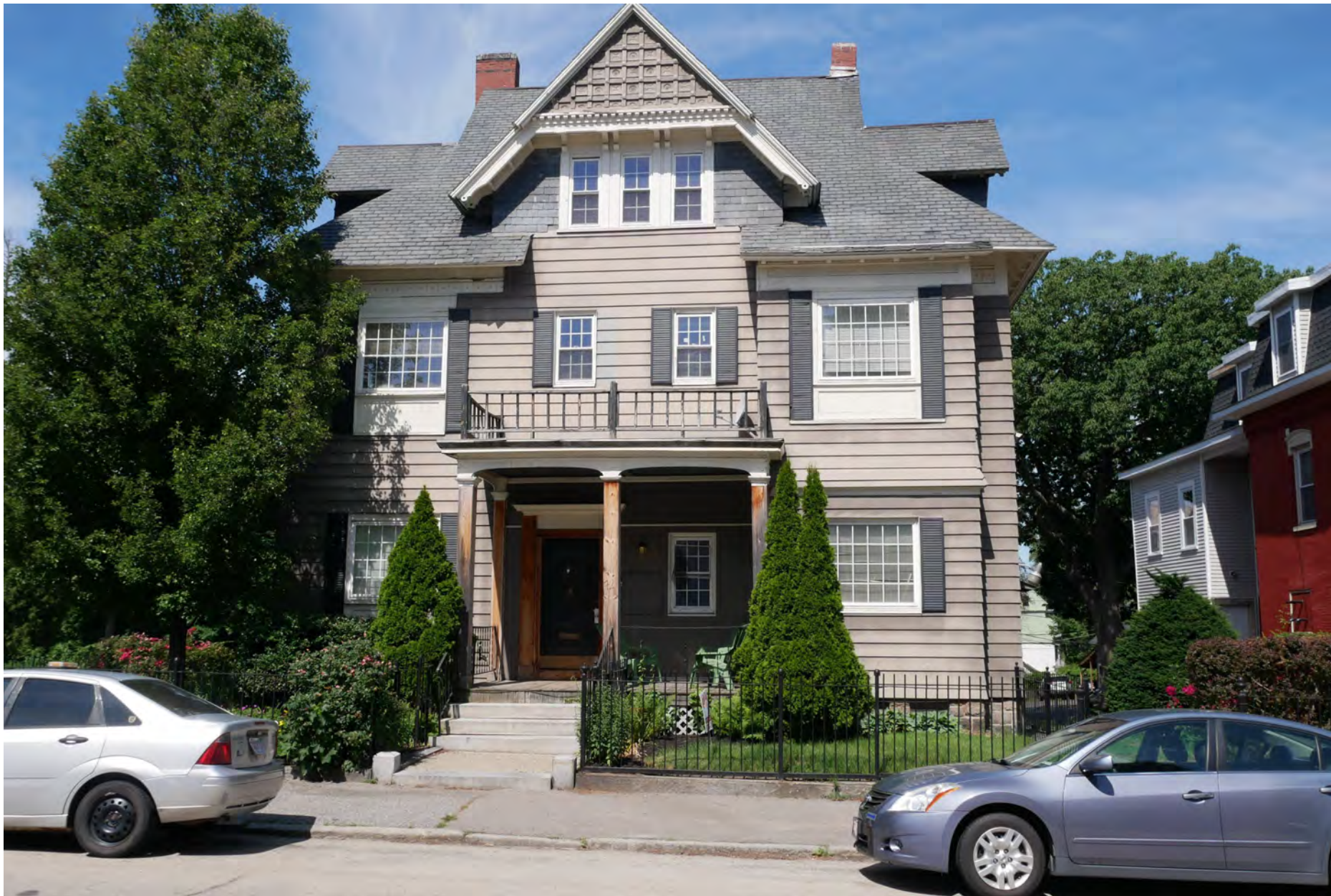
168. 72 West Street, looking west. Integrity rating: fair
