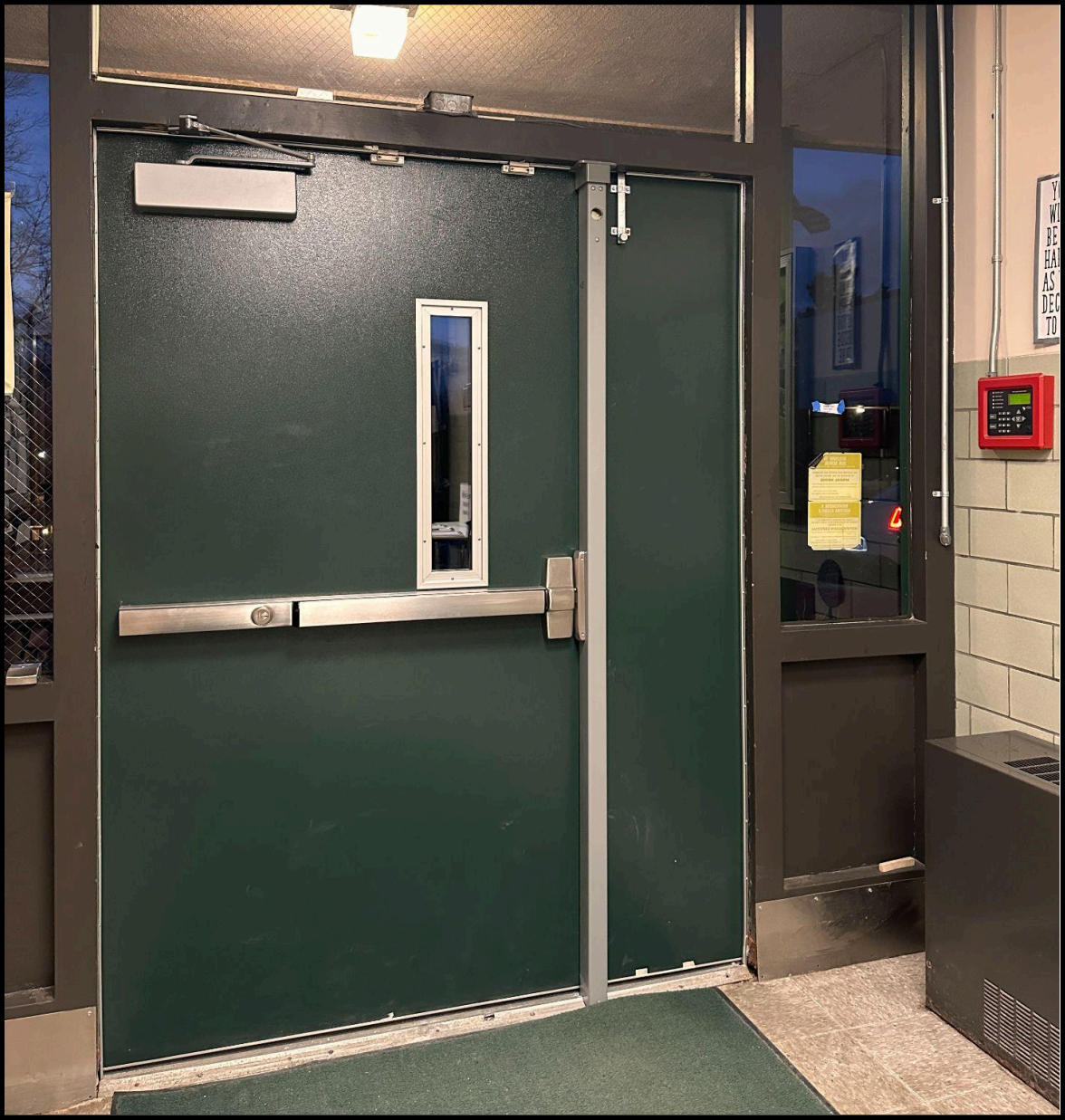
Fig. 6 - Burncoat Middle ADA Upgrades, new ADA compliant main entry door
