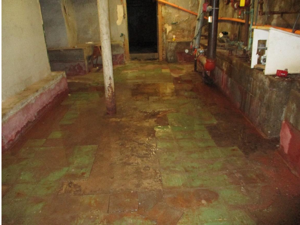
Sample Unfinished Basement
