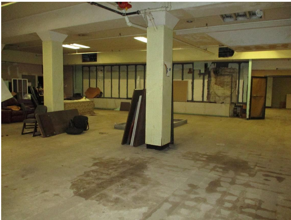
Sample Unfinished Basement
