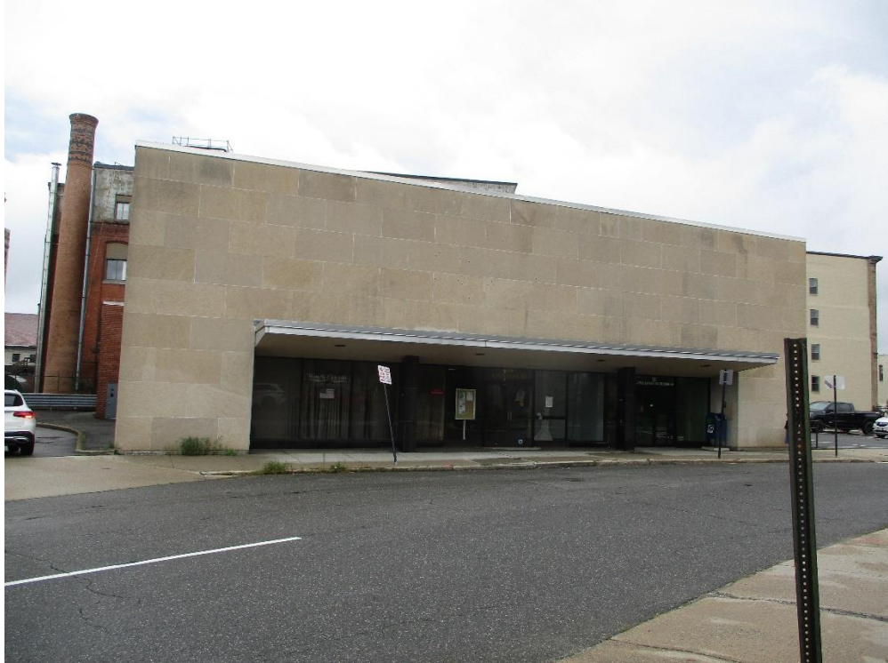
West Side of the Building
