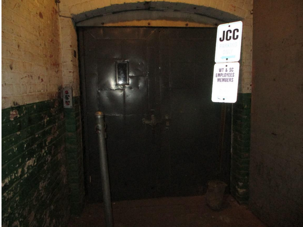
View of Non-Working Freight Elevator
